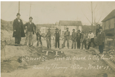
Stewart St. was paved all the way to the city limits in 1909. Thoney Pietro at far right.
